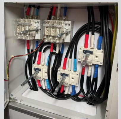
Figure 3: Bypass panel that required detailed inspection during the site survey.
